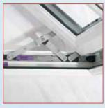
Side hung windows use the Cotswold friction stay - a high quality hinge that allows the entire sash to slide sideways when opened to facilitate the cleaning of the outside of the sash from inside.
